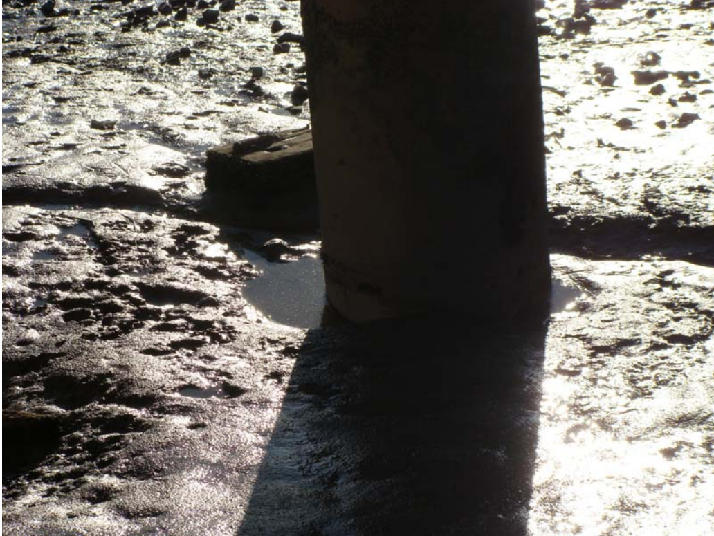
Photo 15. Close-up of pile 1N-A (looking east) – November 21, 2007
