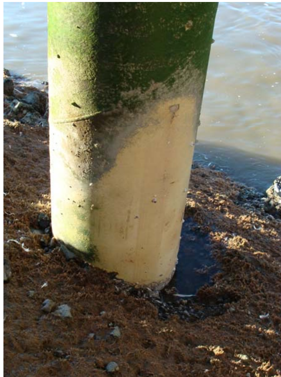
Photo 10. Close-up of pile 1S-A – November 21, 2007
