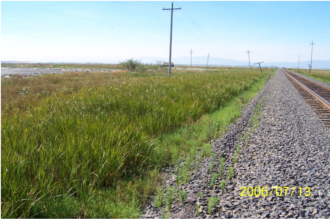
Photo 15. East Rail Levee near Pond A20, view looking south – July 13, 2006.
