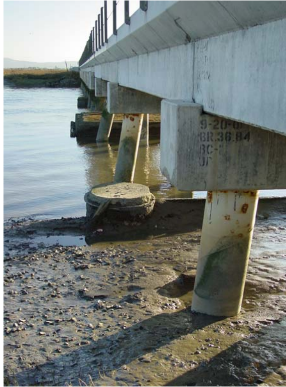
Photo 1. East Side of Bridge Looking South. Pile 1N-C in foreground – November 29, 2006
