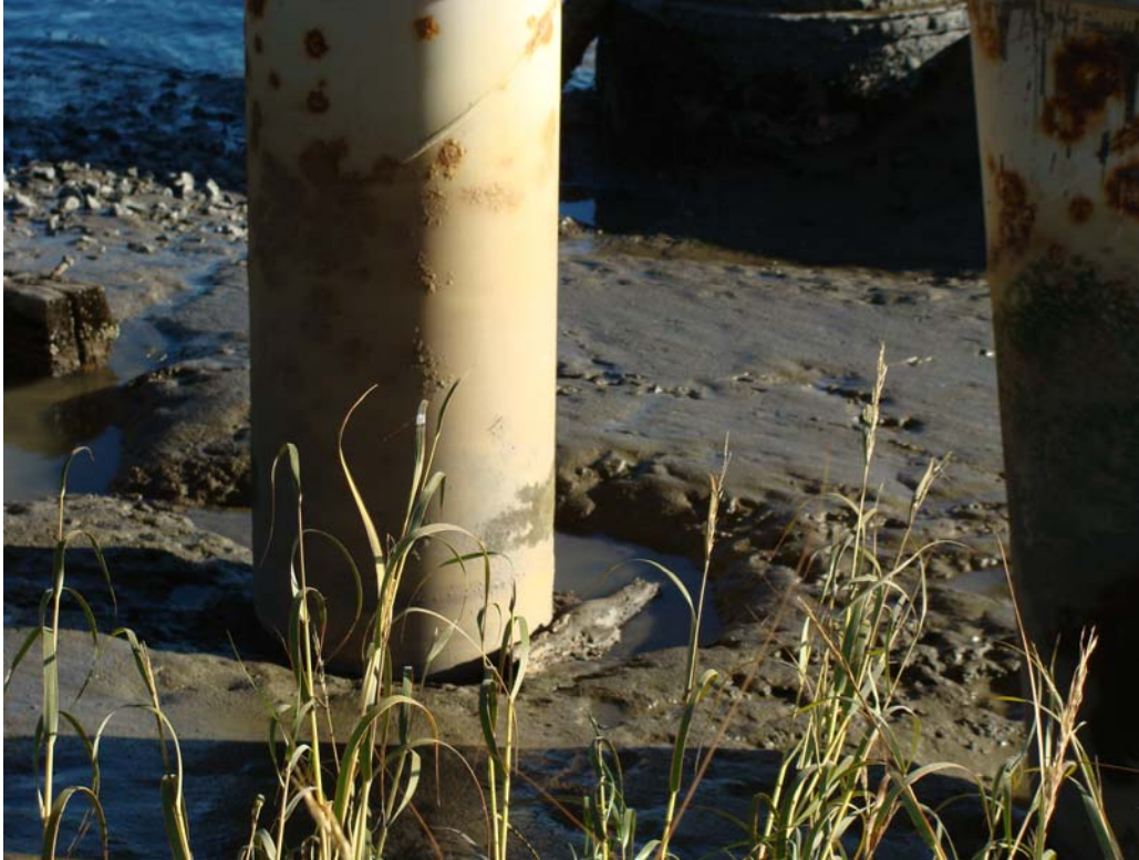
Photo 17. Close-up of pile 1N-B (looking east) – November 21, 2007
