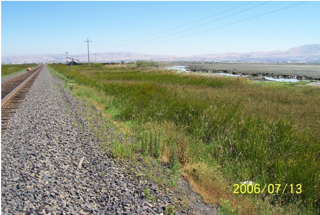
Photo 13. East Rail Levee near Pond A20, view looking north – July 13, 2006.
