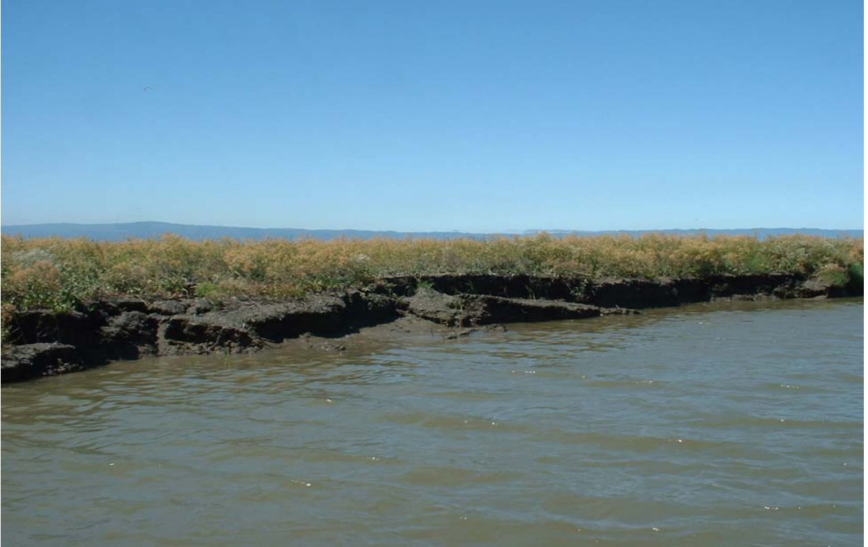
Photo 5: Scour along fringing marsh, southern bank of Coyote Creek – July 24, 2007.
