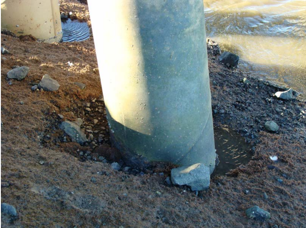
Photo 13. Close-up of pile 1S-C – November 21, 2007
