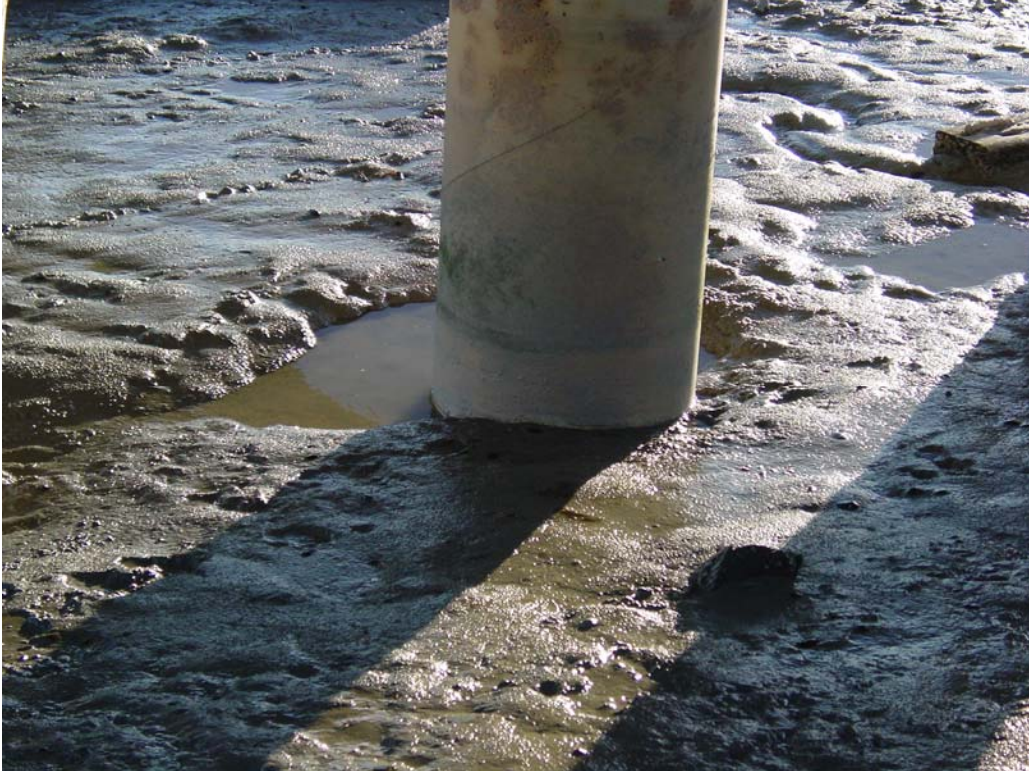
Photo 18. Close-up of pile 1N-B (looking west) – November 29, 2006
