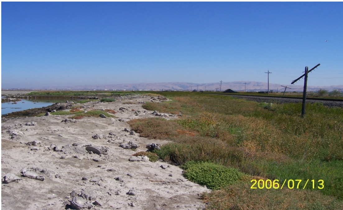
Photo 1. Pond A21 Levee near Rail Levee, view looking north - July 13, 2006.
