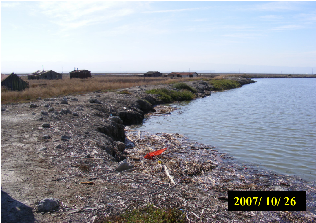
Photo 5. Debris accumulated in the southeast corner of Pond A21. Debris is also visible on top of the levee – October 26, 2007.
