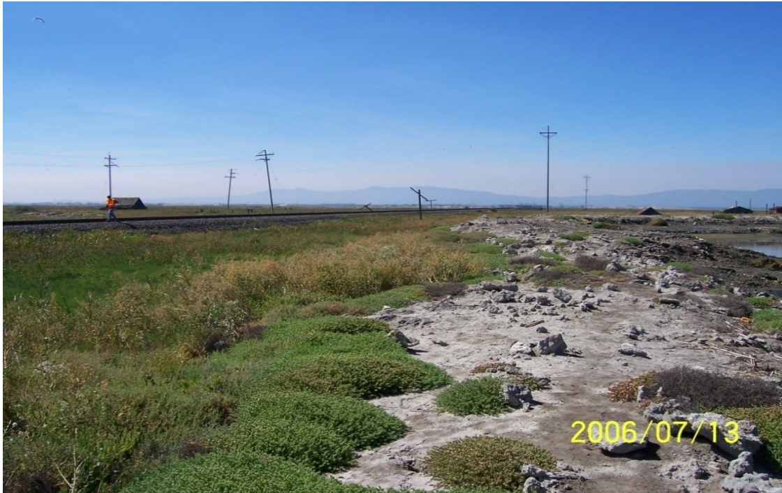
Photo 3. Pond A21 Levee near Rail Levee, view looking south – July 13, 2006.
