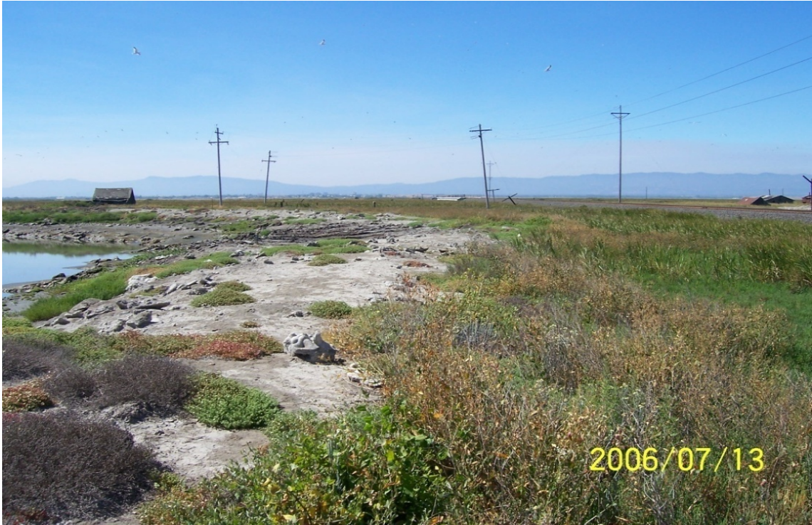
Photo 11. Pond A20 Levee near Rail Levee, view looking south – July 13, 2006.
