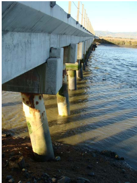
Photo 8. East Side of Bridge Looking North. Pile 1S-C in foreground – November 21, 2007
