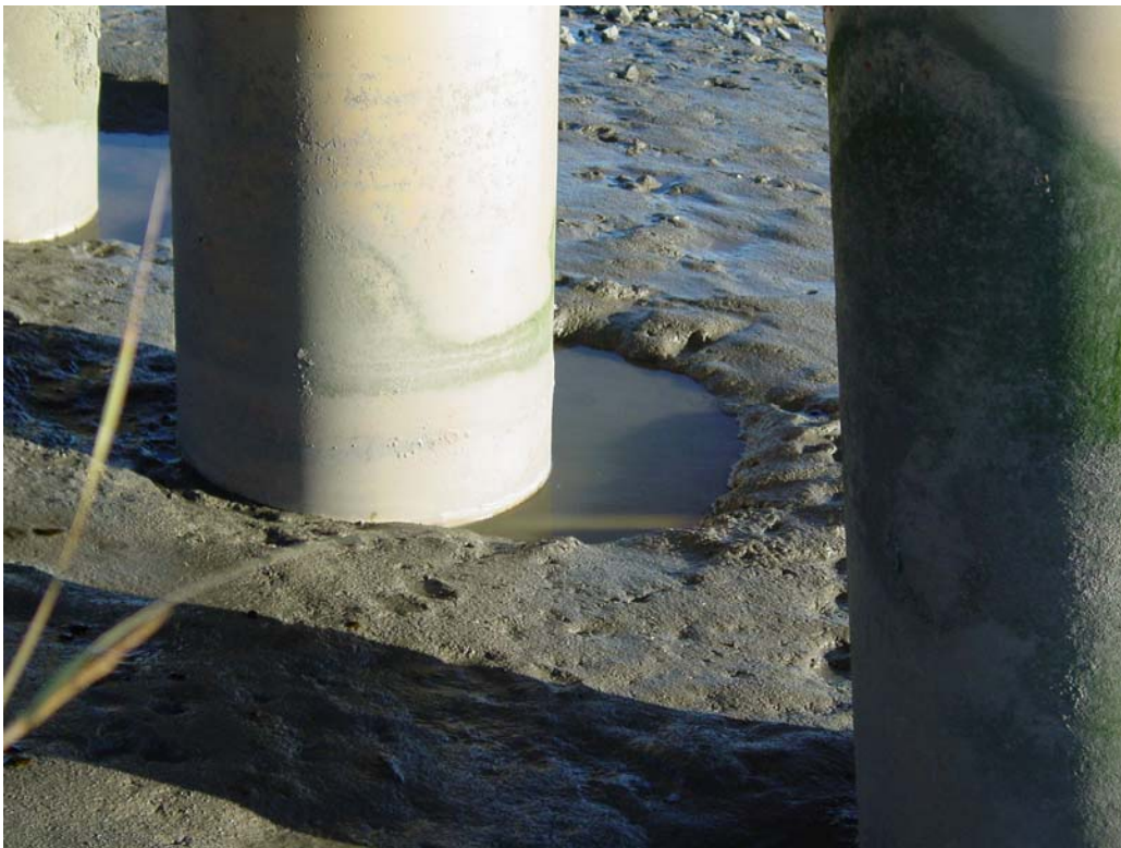
Photo 16. Close-up of pile 1N-B (looking east) – November 29, 2006
