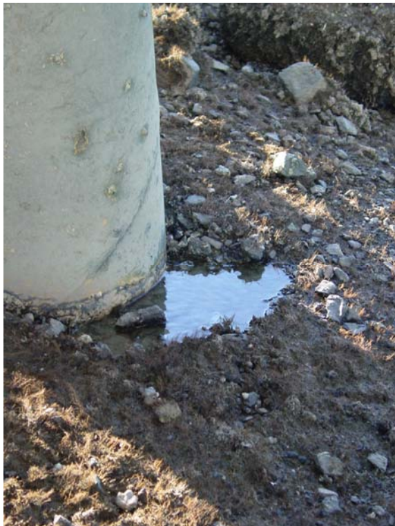
Photo 9. Close-up of pile 1S-A – November 29, 2006
