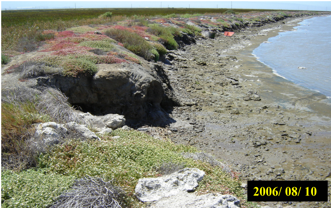
Photo 3. Close up of eroded section of levee in the southeast corner of Pond A21, view looking west – August 10, 2006.
