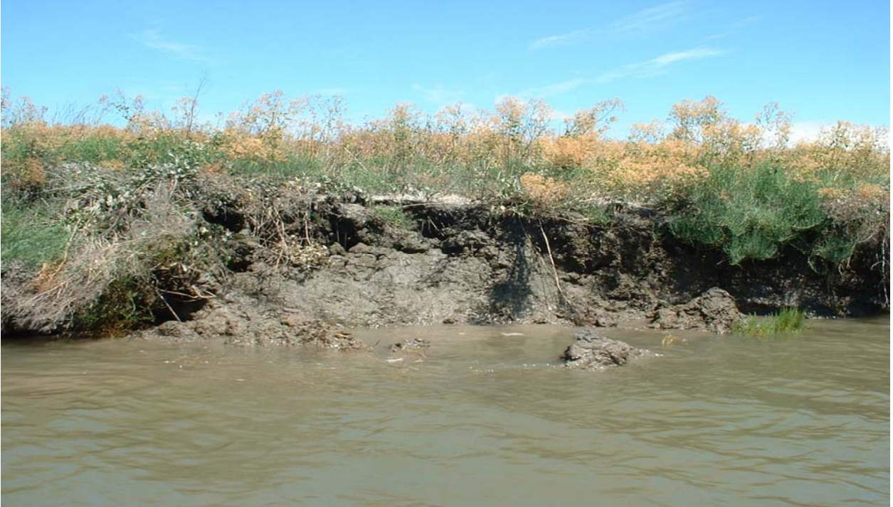
Photo 4. Scour along fringing marsh, southern bank of Coyote Creek – July 24, 2007.
