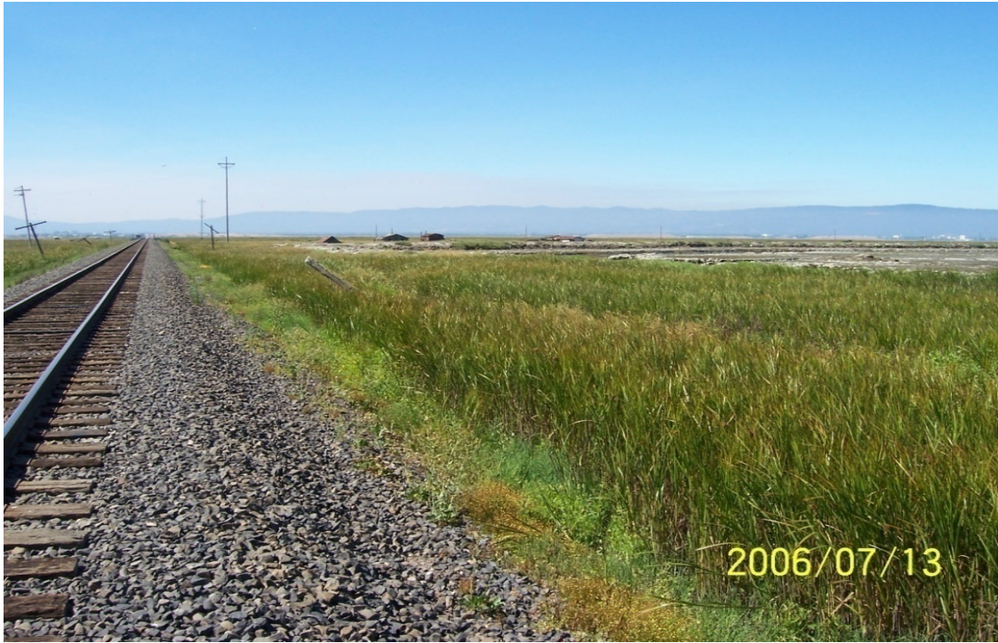
Photo 7. West Rail Levee near Pond A21, view looking south – July 13, 2006.
