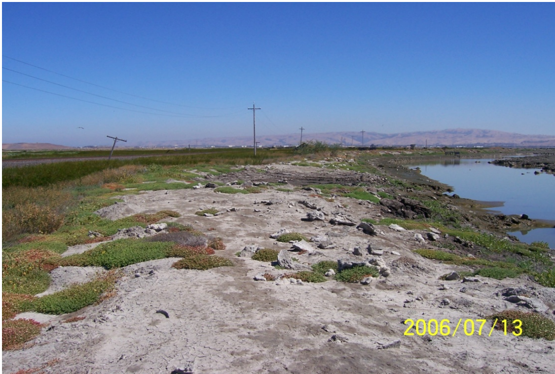
Photo 9. Pond A20 Levee near Rail Levee – July 13, 2007.
