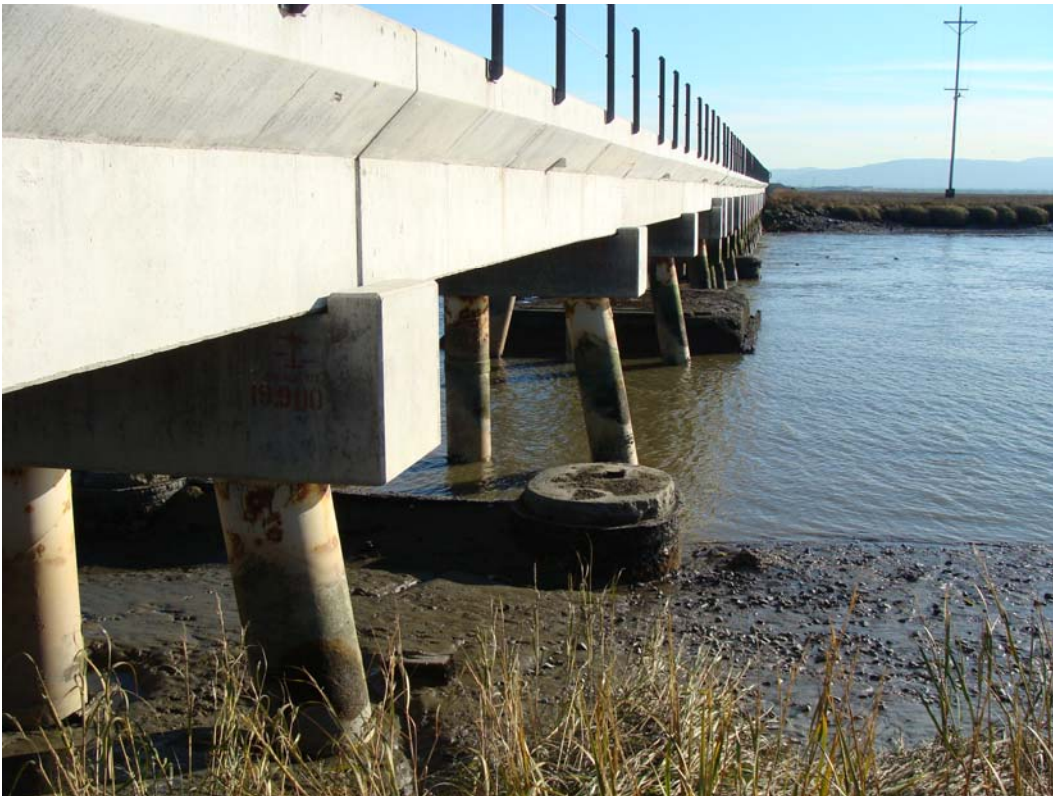
Photo 4. West Side of Bridge Looking South. Pile 1N-A in foreground – November 21, 2007
