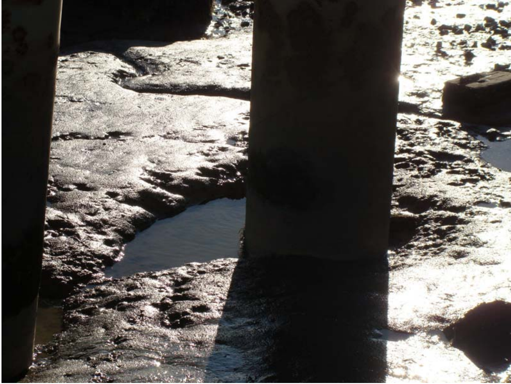
Photo 19. Close-up of pile 1N-B (looking west) – November 21, 2007
