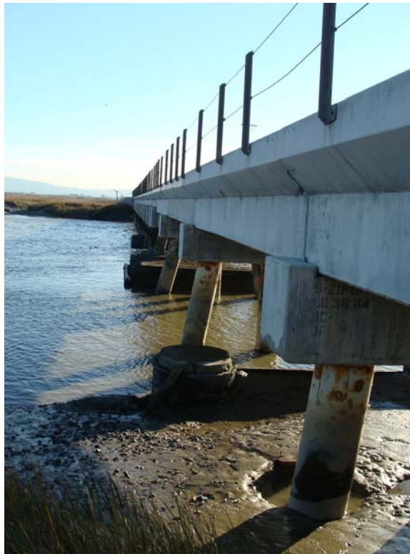
Photo 2. East Side of Bridge Looking South. Pile 1N-C in foreground – November 21, 2007
