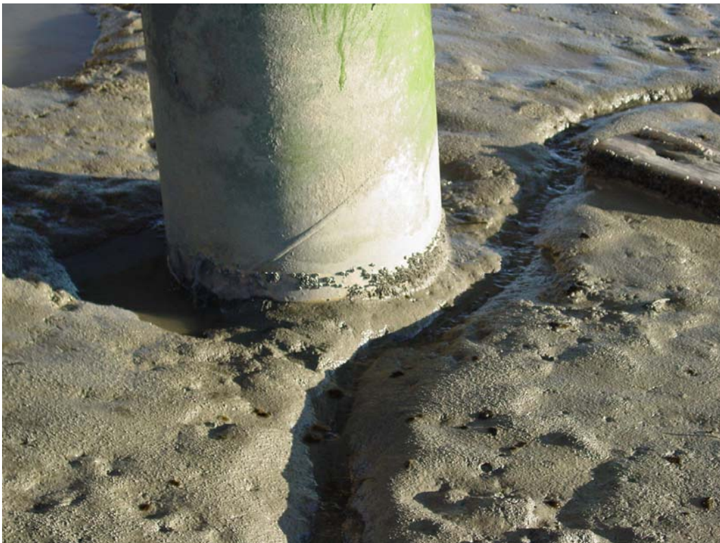
Photo 14. Close-up of pile 1N-A (looking west) – November 29, 2006
