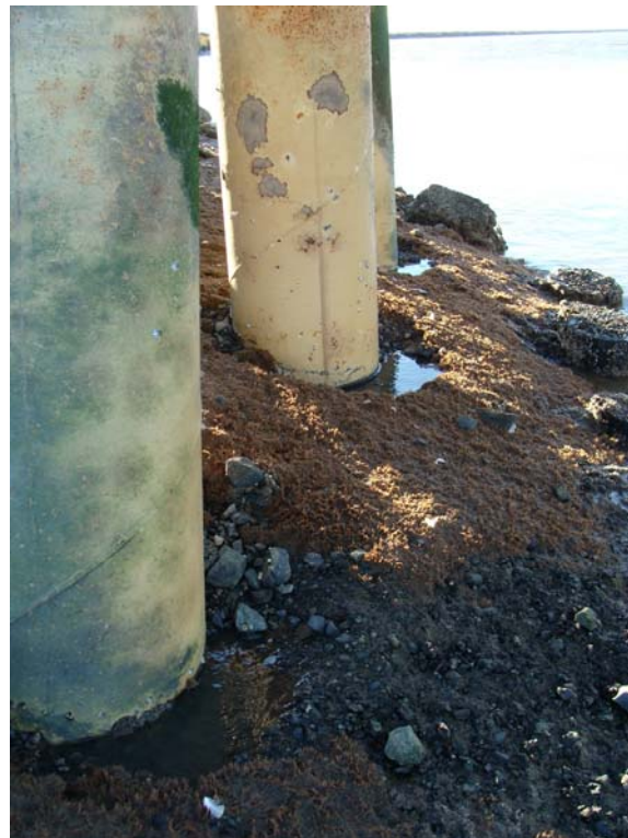
Photo 12. Close-up of piles 1S-C (foreground), 1S-B (centre), and 1S-A – November 21, 2007
