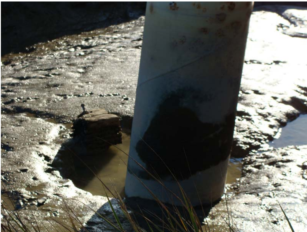
Photo 20. Close-up of pile 1N-C – November 29, 2006
