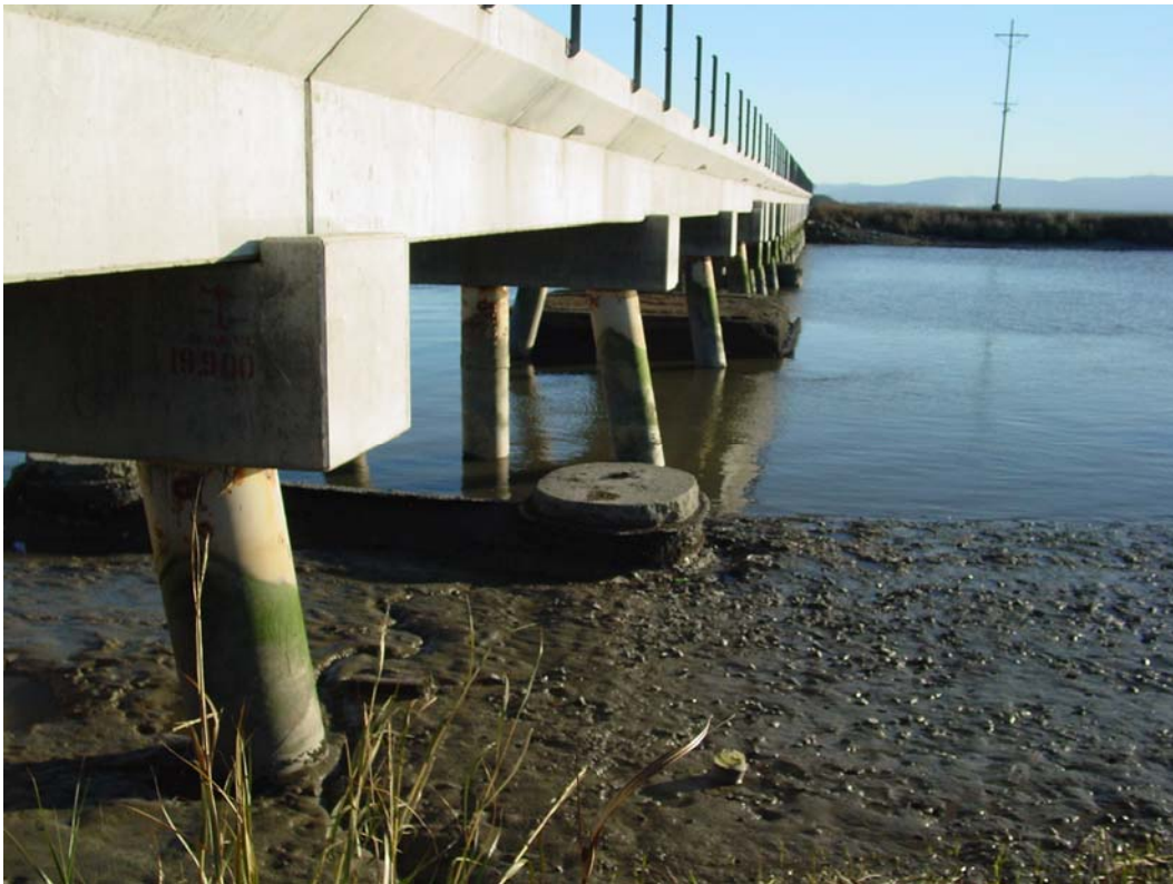
Photo 3. West Side of Bridge Looking South. Pile 1N-A in foreground – November 29, 2006
