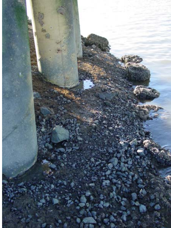
Photo 11. Close-up of piles 1S-C (foreground), 1S-B (centre), and 1S-A – November 29, 2006
