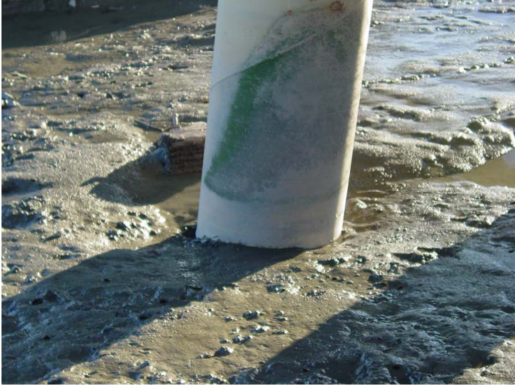
Photo 21. Close-up of pile 1N-C – November 21, 2007
