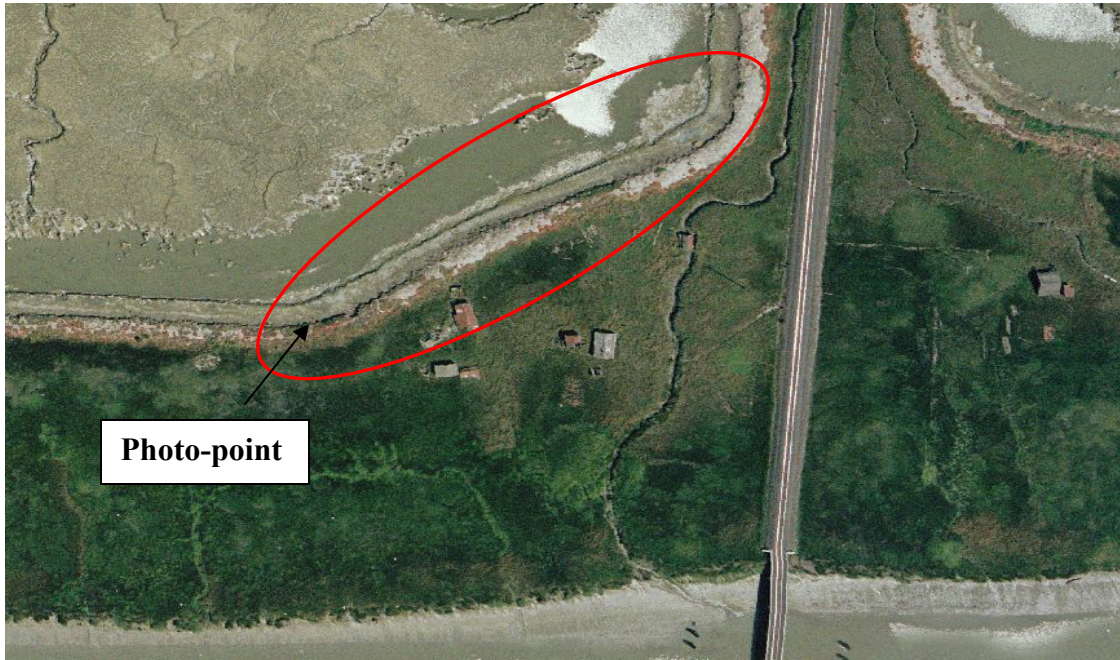
Photo 1. Aerial view of railroad and Town of Drawbridge. The red circle (southeast levee of Pond A21) depicts the area which is eroding.
