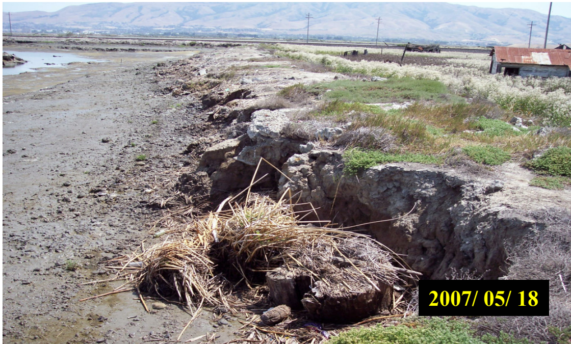
Photo 2. Levee erosion at Pond A21's southeast levee, view looking east – May 18, 2007.
