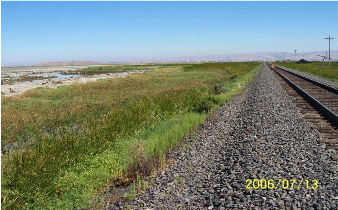
Photo 5. West Rail Levee neat Pond A21, view looking north – July 13, 2006.
